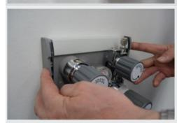
Step 5. Insert the plastic side sections into the basic profile.
