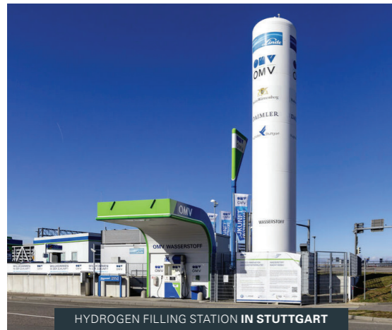
HYDROGEN FILLING STATION IN STUTTART
